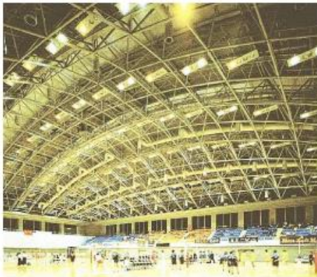
Figure 13. Tokuyama multipurpose hall Taiyo Kogyo TM-System (Design, Analysis and Construction of space Structure, the Mero Legacy)
